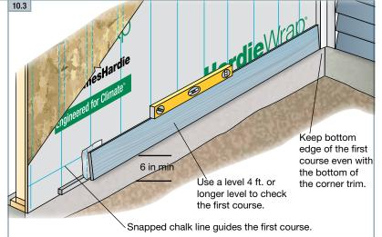
odically check the level and straightness of the courses. When correcting for flatness over products such as exterior insulation, use drywall shims. It is good practice to snap a chalk line every 3 to 5 courses to keep the planks straight and level.
