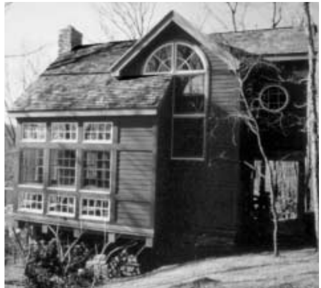
Figure 10. Corner Boards
